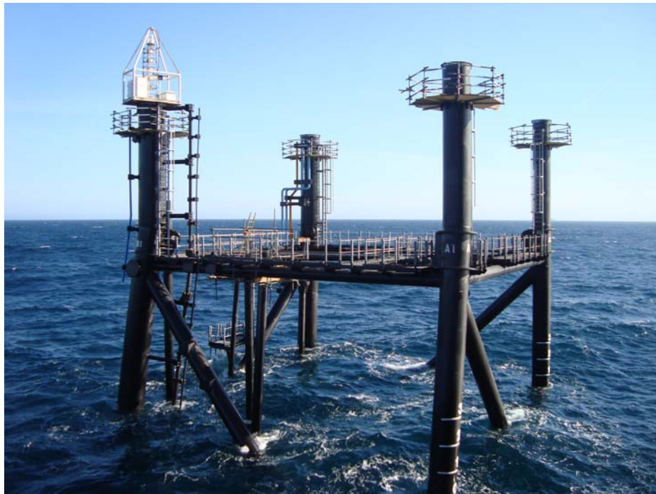
A package of Tideland aids to navigation installed on the jacket of a new platform for GDF SUEZ E&P Nederland BV in the Dutch sector of the North Sea. Picture courtesy of Seaway Heavy Lifting / GDF SUEZ E&P Nederland B.V.
